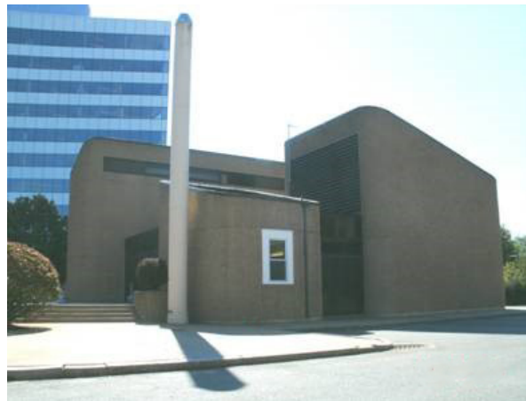
Prison Point CSO Facility – Main Building
