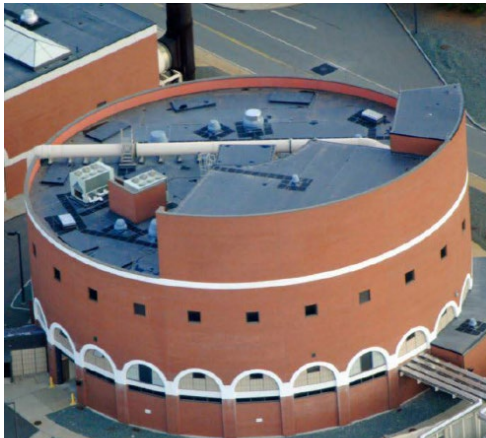
South System Pump Station
