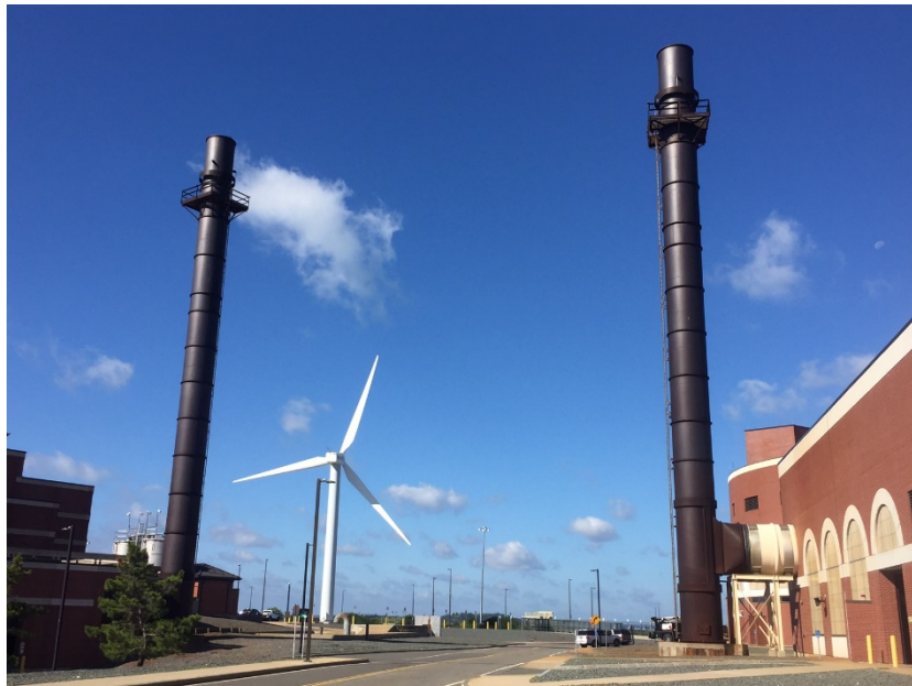
Deer Island Odor Control Emission Stacks
